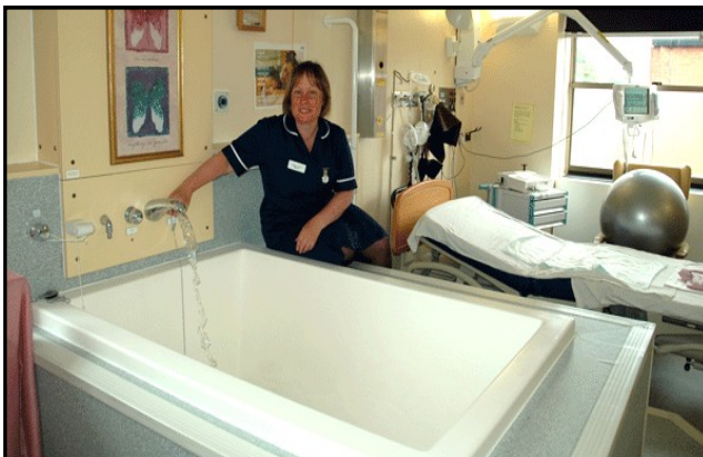
An example of a plumbed-in birthing pool
